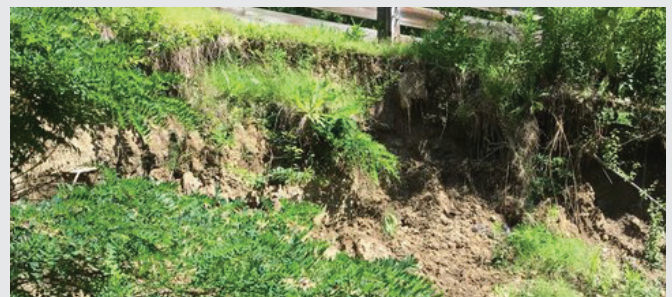
Muddy Creek before restoration and protection
