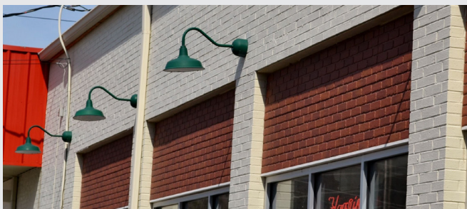
Goose Neck lighting from the building
