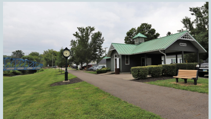
Renovated historic train depot on the B&O Trail in Bellville, OH
