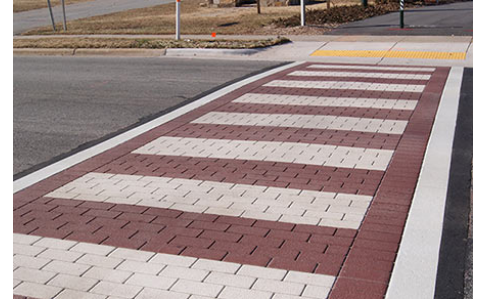
A crosswalk on W Market St provides an active transportation route to the River while promoting safe and accessible options.
